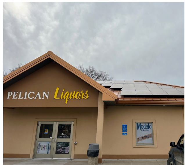
Photo: Solar array on Pelican Rapids municipal liquor store.
